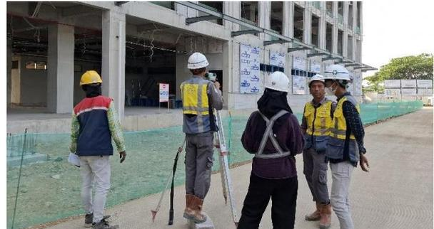
**Gambar 2. Pengukuran Settlement Gedung X**
